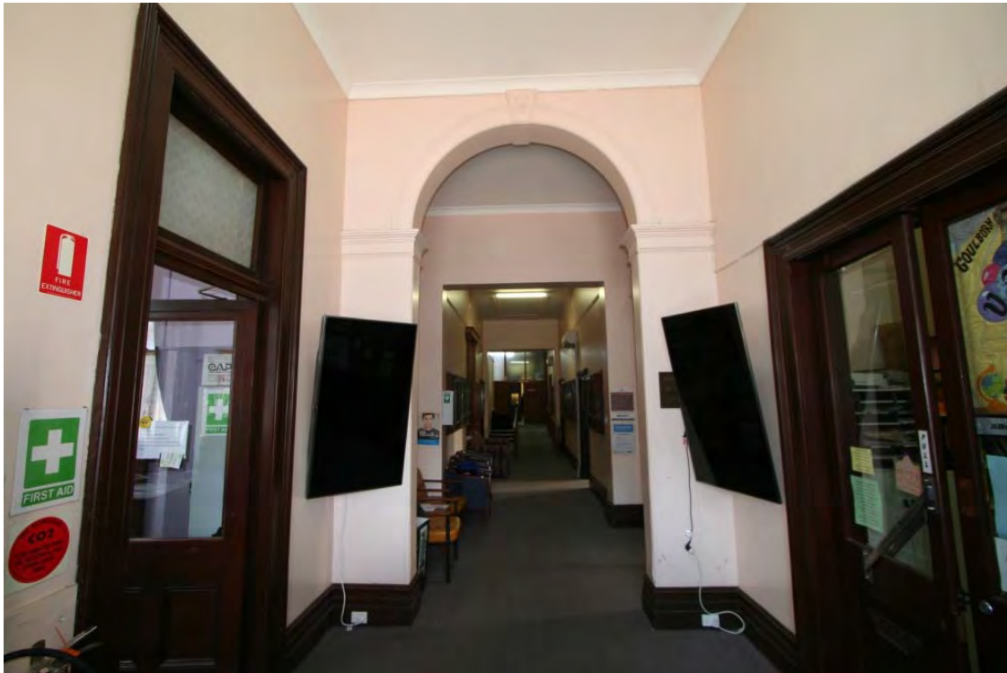
Photograph 17 View from the entry illustrating the original arch separating the lobby from the second opening. The original walls and doors to the left (minor offices) and right (major office) are to be demolished.
